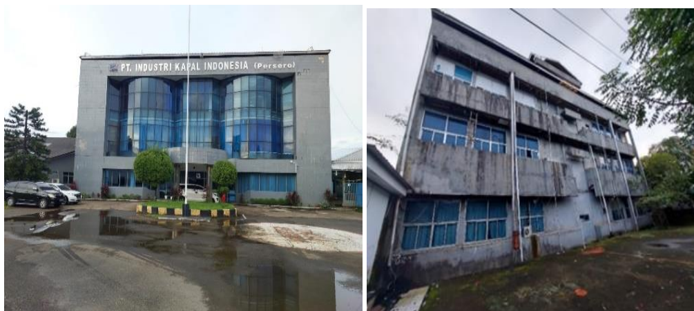
Figure 2. PT. IKI Building Façade
