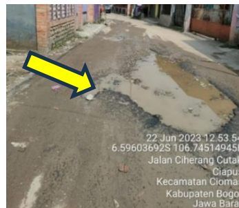
Figure 5. Holes 0+300 - 0+400. Source: Research data
