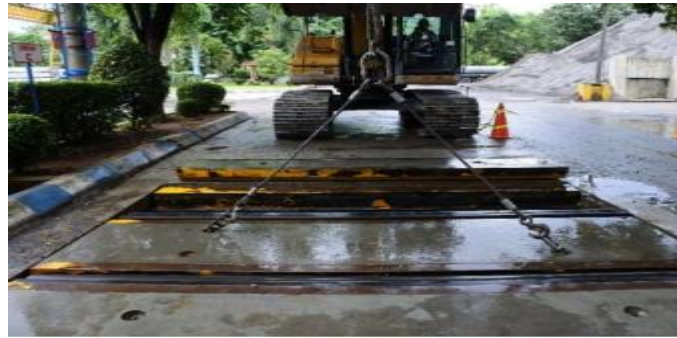
Figure 19. Lifting and Stacking CLC Plate Source: Wika Beton Handling Manual
