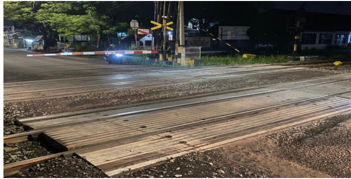
Figure 4. Railway level crossing with CLC. Source: Personal Documentation
