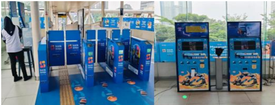
Figure 6. Automatic Tapping Door and Vending Machine (Source: Personal photo, 2023)
