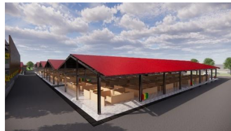
e. Block D building with an area of 864 m 2
