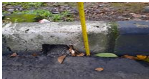
Figure 3. Sidewalk height Source: personal documentation 2025
