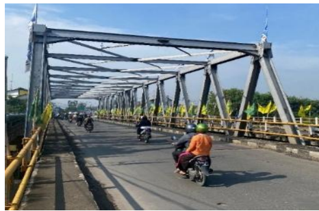
Figure 1. Citarum Baru Bridge
