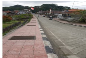
Rainwater channel network for local flood control/ drainage and prevention
