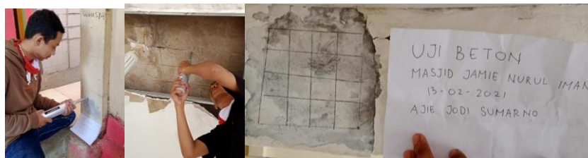
Figure 5. Testing the quality of concrete. Source: Personal documentation
