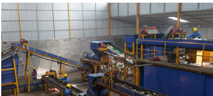
Figure 4. Segregation of Waste at TPST Samtaku – Jimbaran. Source: https://www.reciki.co.id
