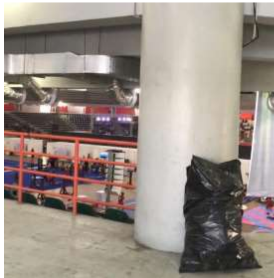
Figure 2. Plastic waste inside the multipurpose building
