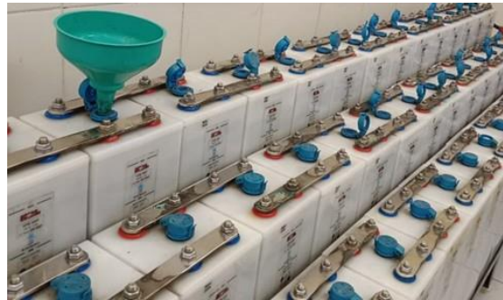
Gambar 3. baterai 110Vdc Unit 1 GI Bogor Baru
