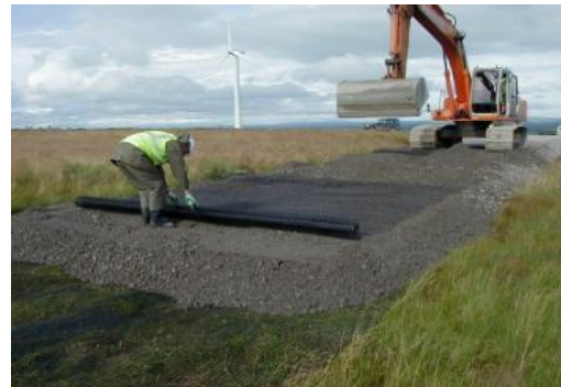
Figure 3: Stabilized clay soil with geotextile Source: Engineering Daily, 2023
